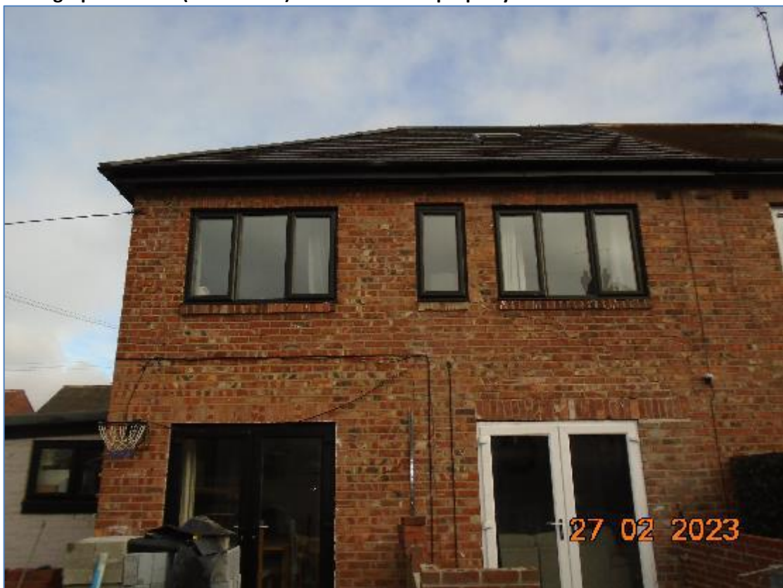
Photograph 2 – Rear (south-west) elevation of the property.
