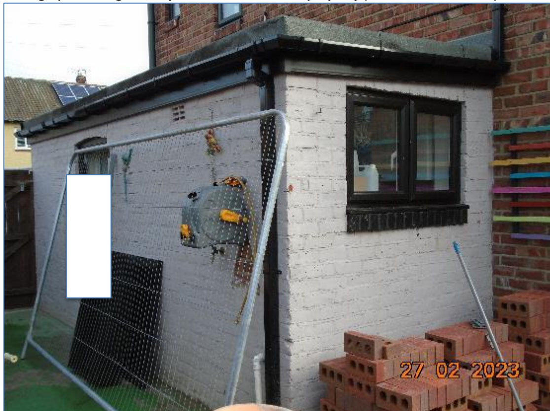
Photograph 4 – Single storey side extension to the property (north-west elevation).
