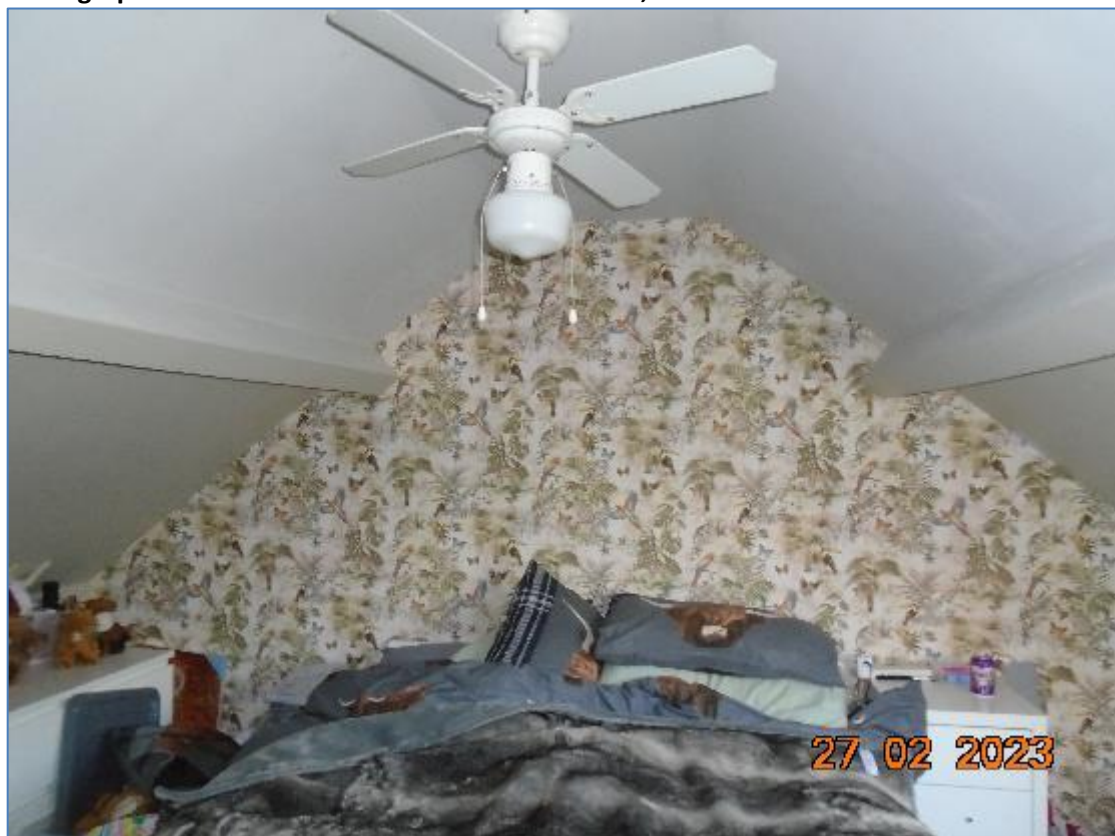
Photograph 6 – Interior view of the former roof void, now converted for habitable use.
