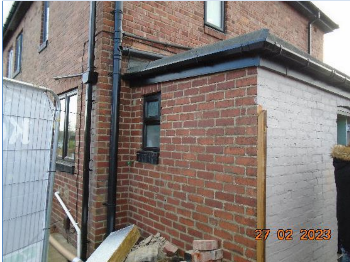
Photograph 5 – Close fitting fascia boards on the single storey side extension.
